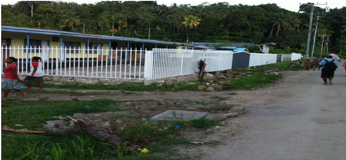
Figure 1: PCDF fencing project of Kirakira Hospital, December 2012
